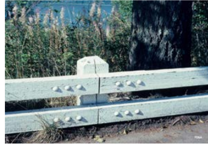
Top left: New section of the Historic Columbia River Highway State Trail at Shell Rock, 2018. Courtesy: Oregon Department of Transportation.
