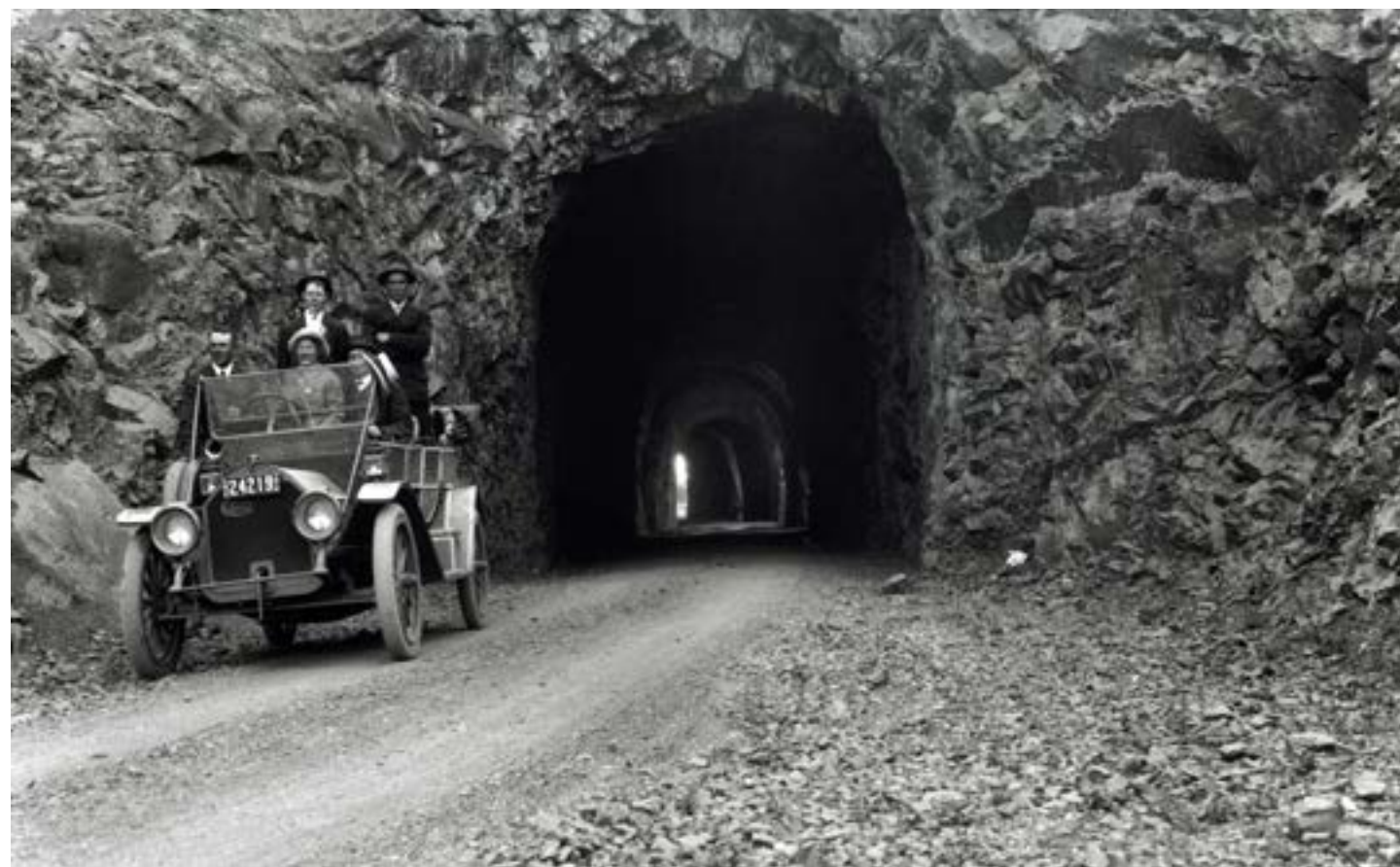
Mitchell Point Tunnel, east entrance. Courtesy: Oregon Department of Transportation.
