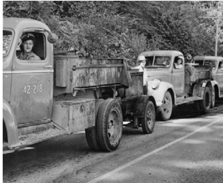
Women's WW II Paving Crew, 1934. Courtesy of Oregon Department of Transportation.
